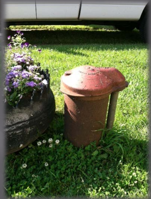
Water Supply Well
