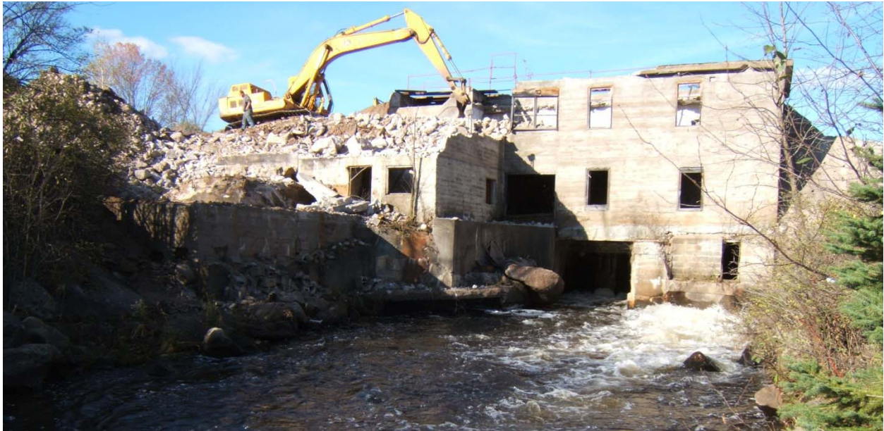
Figure 1. Grimh Dam powerhouse during removal
