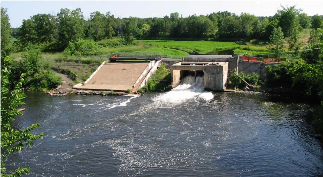
Figure 3. Woodley Dam before removal
