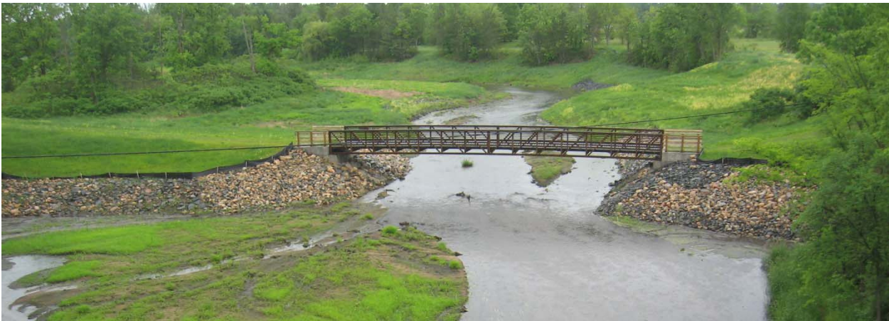
Figure 4. Woodley Dam after removal
