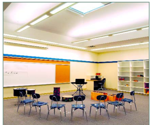
Skylights in the music room, in the central core of the building, exemplify a way in which natural lighting is used throughout the school.
