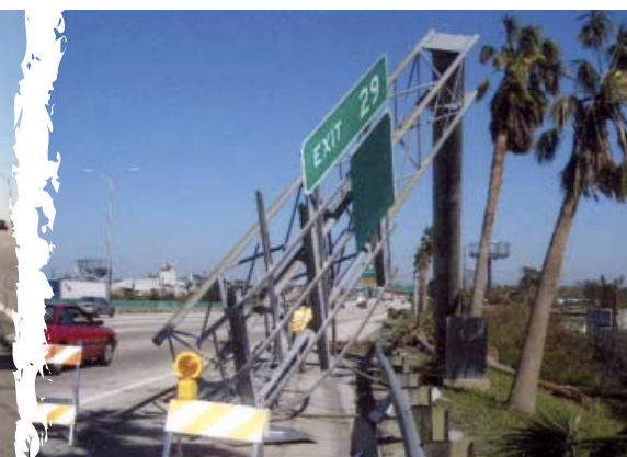
Battered bridges, culverts, and overhead signs in southeast Florida were carefully inspected after Hurricanes Katrina and Wilma.
