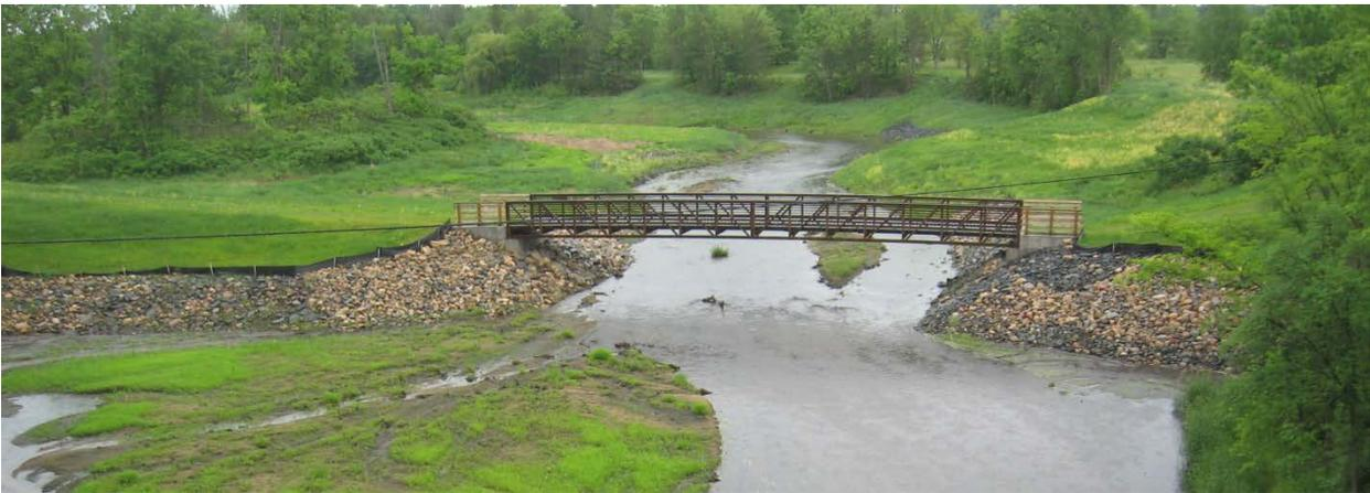
**Figure 4.** Woodley Dam after removal
