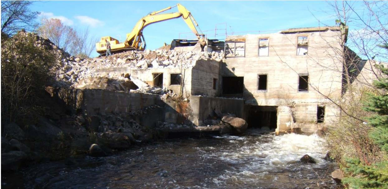
**Figure 1.** Grimh Dam powerhouse during removal
